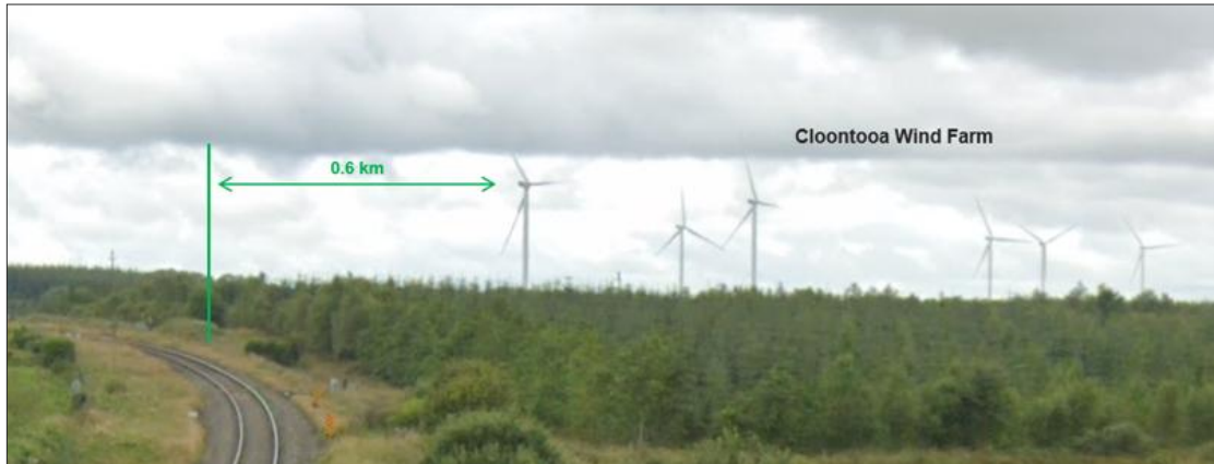
Figure 16. Cloontooa wind turbines shown relative to Irish Rail track
