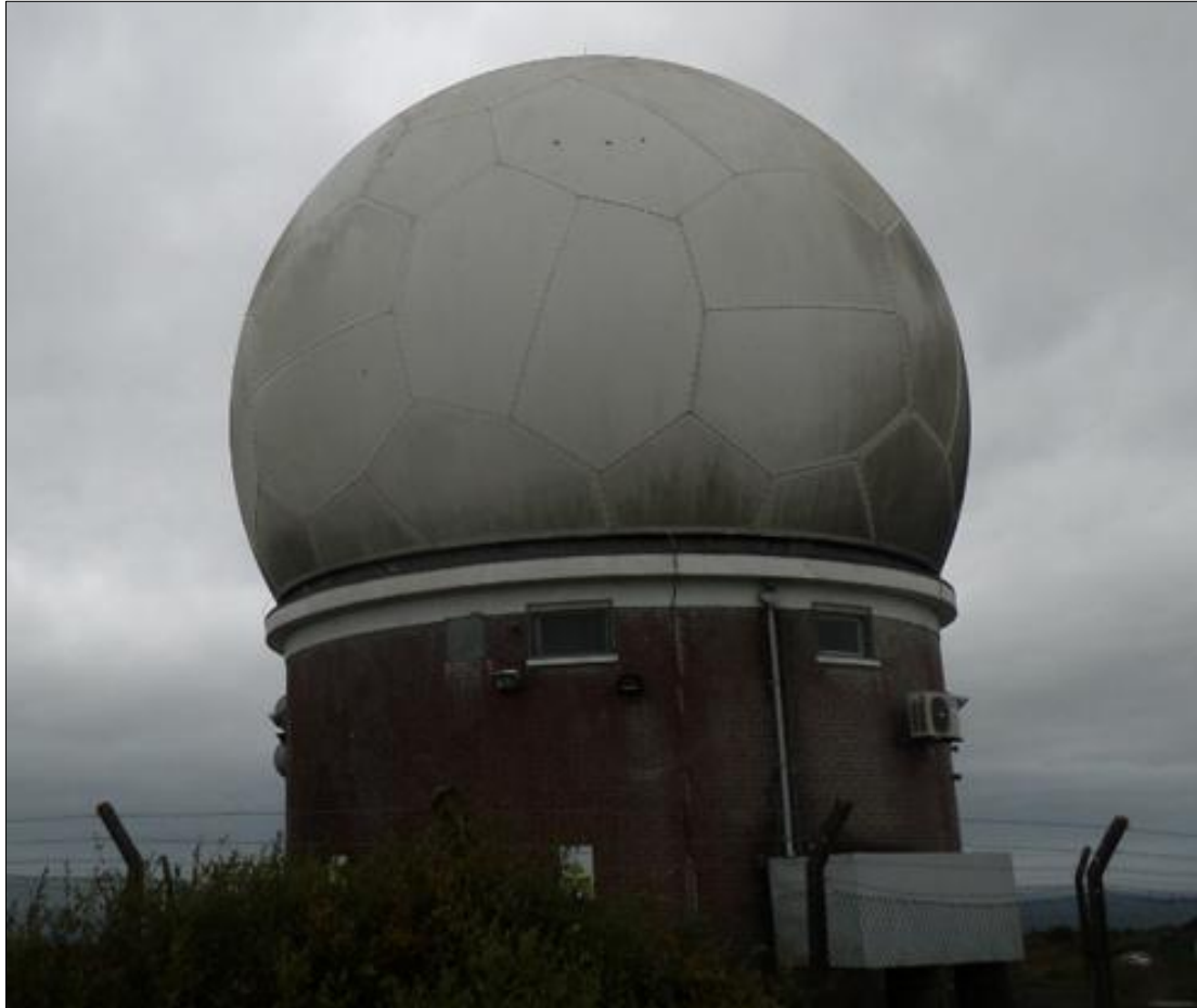
Figure 12. Woodcock Hill Radar Station
