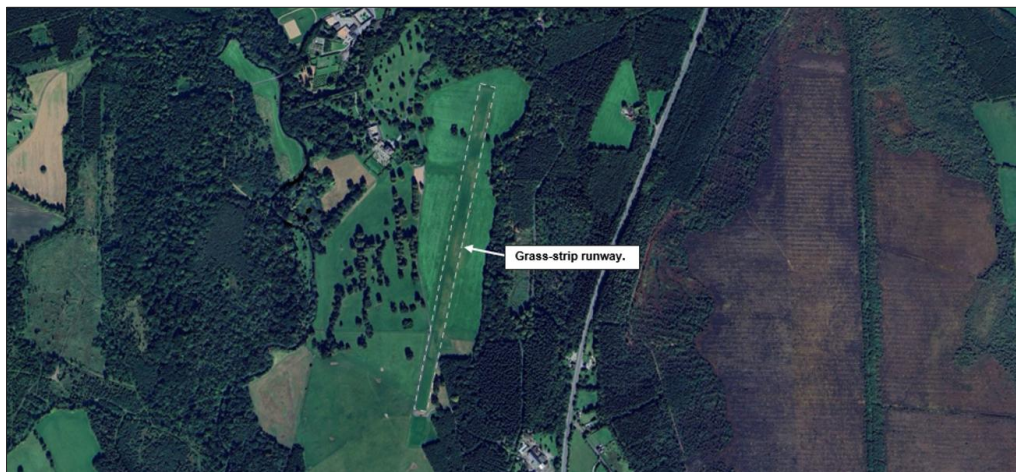
Figure 24. Close-up Aerial View – Abbeyleix Airfield
